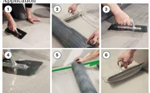
Apply Aquastop Nanoflex with a smooth spreader in thicknesses of about 1 – 2 mm, pressing down to ensure maximum adhesion to the substrate. The resulting thickness depends on the surface finish and on the irregularity of the substrate.
