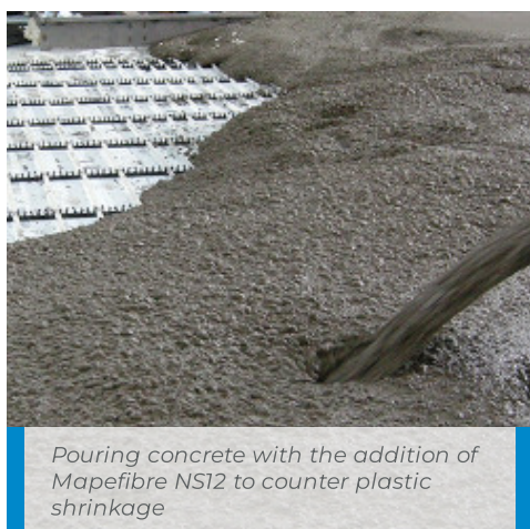
Example of industrial flooring admixed with Mapefibre NS12
