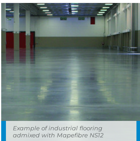
Pouring concrete with the addition of Mapefibre NS12 to counter plastic shrinkage
