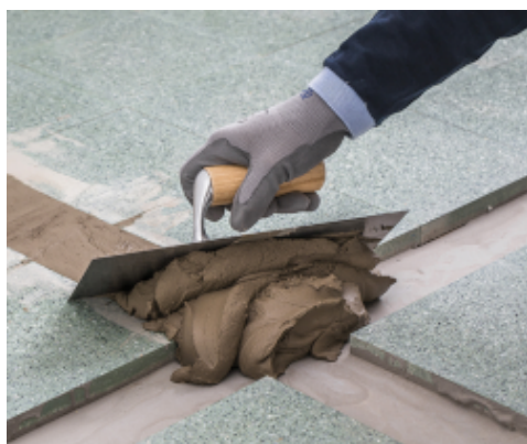
Filling a cable run with Planipatch Xtra
