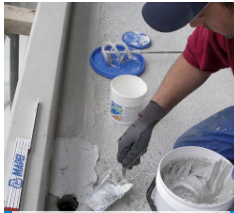
Applying Adesilex PG4 with a trowel
