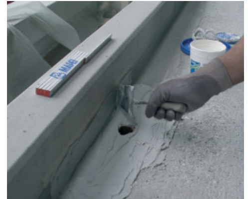
Final covering with Adesilex PG4
