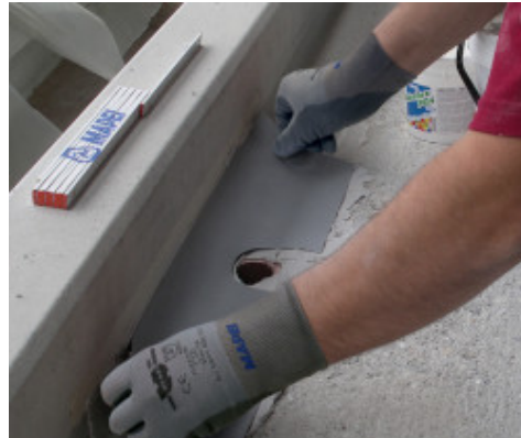
Laying flexible hyphalon brace
