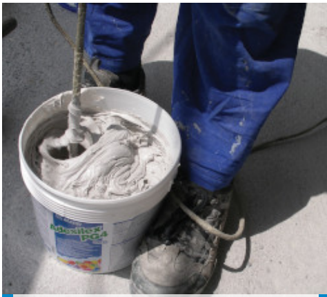
Preparing the mix
