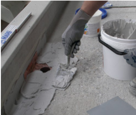
Subsequent smoothing with Adesilex PG4
