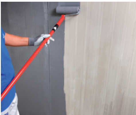
Application of Eco Prim Grip Plus on concrete by roller
